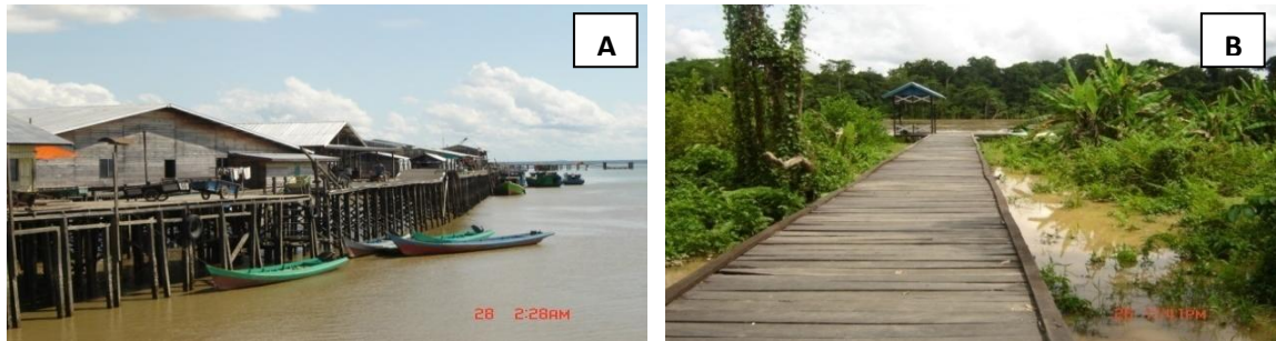
Figure 2. (A) House in coastal area of Balikpapan above water with ironwood pillars and posts; (B) Footpath or bridge made from ironwood timber
