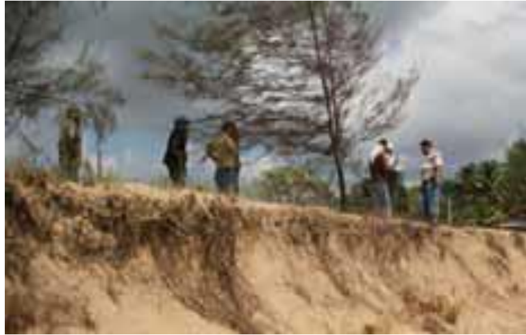
Photo 4. Coastal deterioration (Photo courtesy of Forest Department, 2011)
