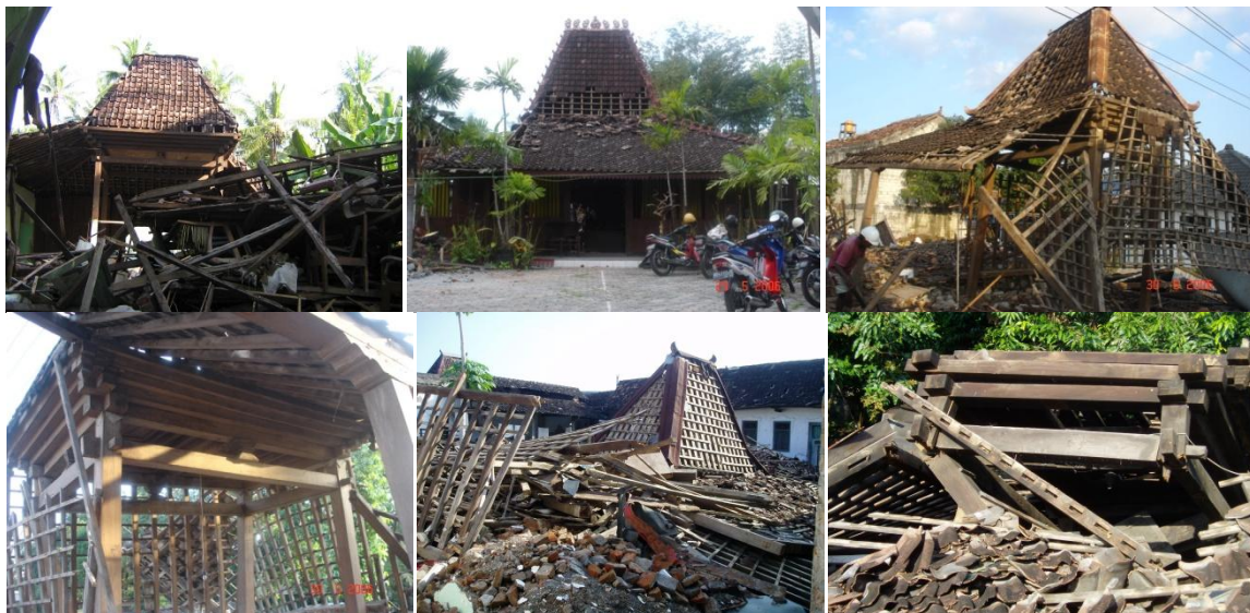
Figure 1. Some Joglos are damage and collapse by Yogyakarta earthquake Source: Prihatmaji, 2006.
